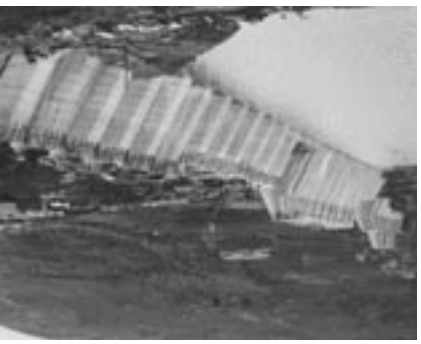
Haweswater Dam under construction in 1930
